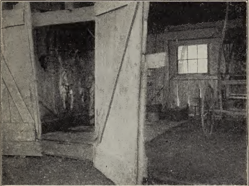
FIG. 3.—Interior of house shown in figure 2.
